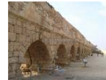
The aquaduct at Caesarea by the sea
